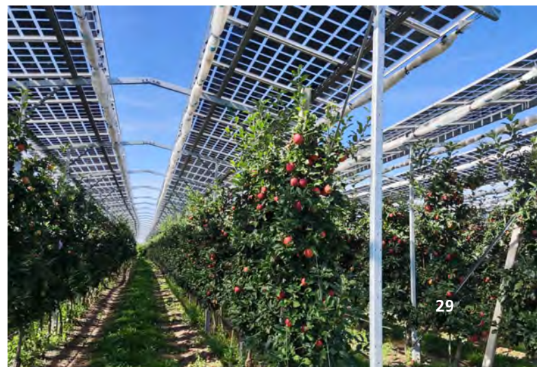
Abb. 28: Agri-PV-Anlage in Kressbronn (2022) © Fraunhofer ISE
